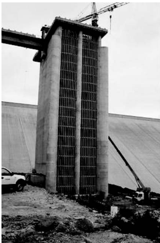
Figure 3.1. Berg Dam 63 m high intake structure upstream of the dam
